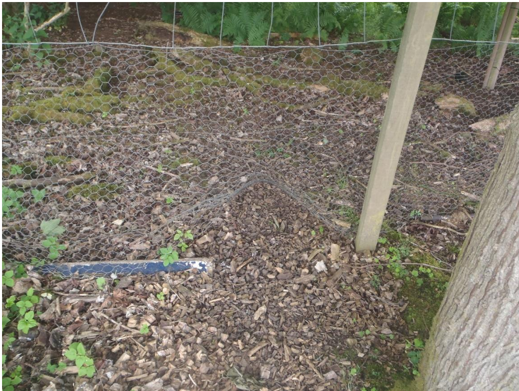
Photograph 4: showing a hole in the boundary fence
