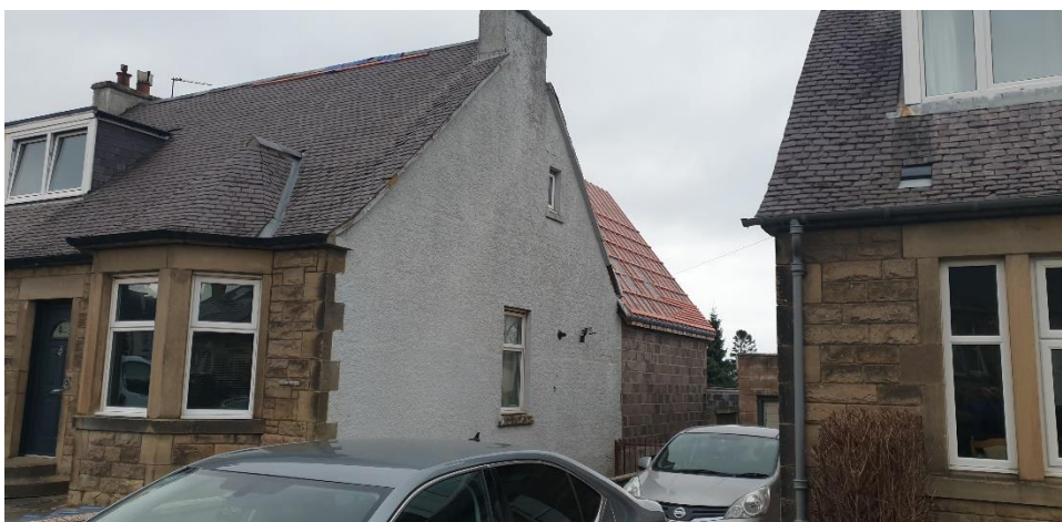
Above is 20 Corbiehill Ave (extension of our clients street) - large rear extension with gable end.
