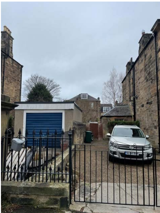
Figure 6 - View of upvc windows at the back of Mayfield Gardens viewed from Glenorchy Terrace.
