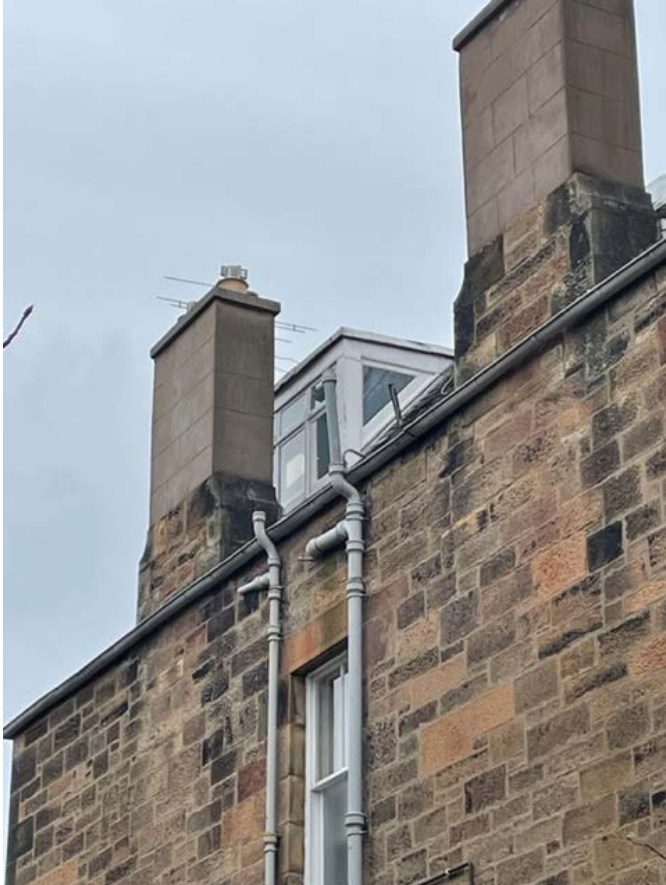
Figure 5 - 3 Glenorchy Terrace - high level upvc window opposite number 4.
