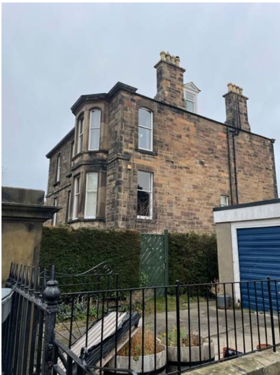
Figure 4 - Side view of corner villa. Upvc windows.
