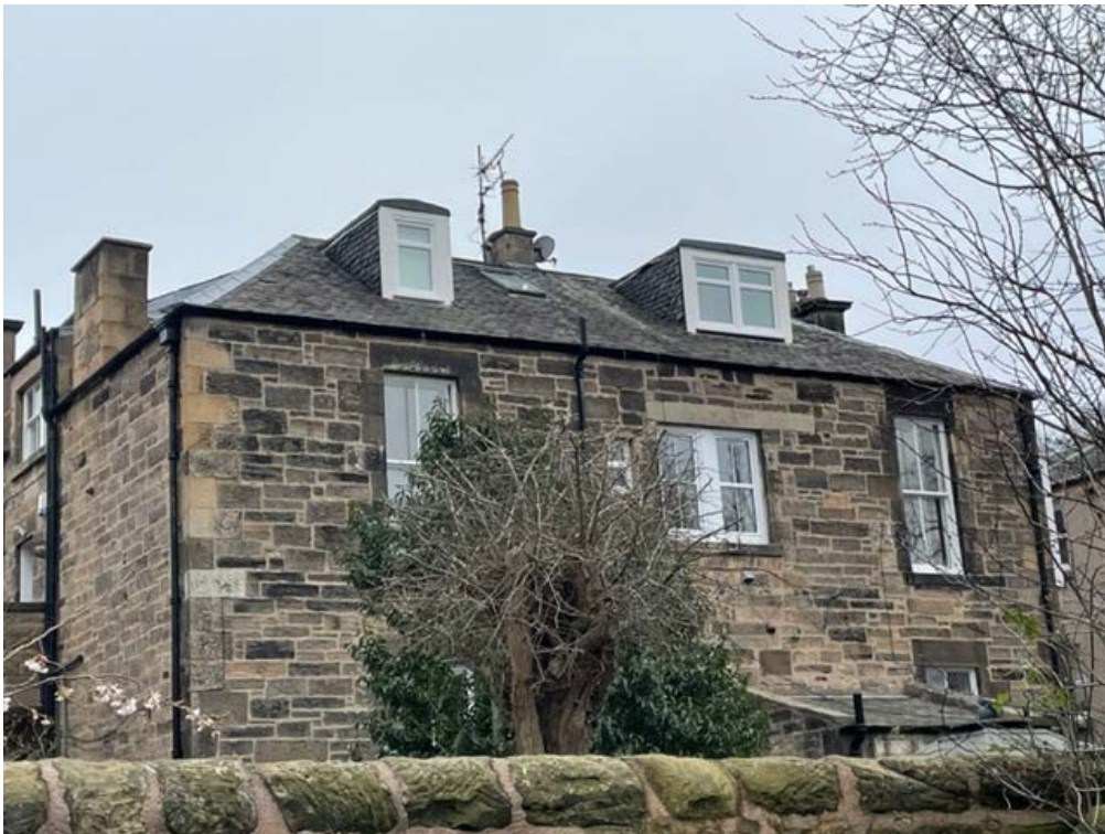
Figure 8 - 14 Mayfield Gardens - upvc windows that can be viewed between villas from Glenorchy Terrace.
