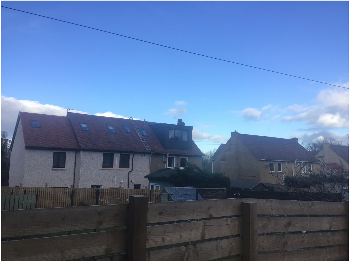
Rear dormer at 40 Station Road taken from 8 Queen Margaret Drive.
