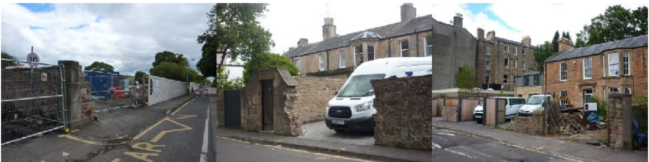
Canaan Lane recent developments and modifications to historic walls.
